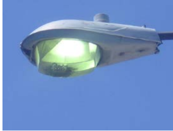
Figure 11 : 175 Watts Mercury Vapor - South Boston, Boston, Massachusetts 37
